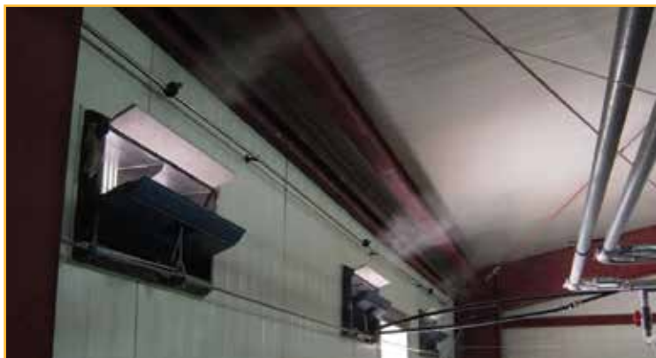
Figure 118: Example fogging system for a cross-ventilated house.
