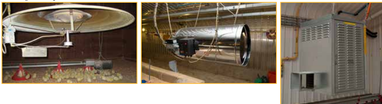
Figure 98: Examples of different house heating systems (from left to right, canopy brooder, whole-house heating, and space heater).
