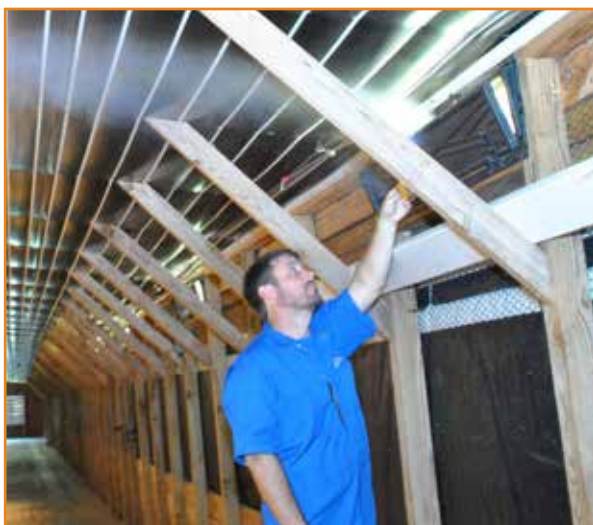
Figure 6.7: Using a smoke test to determine if airflow and operating pressure is correct.
