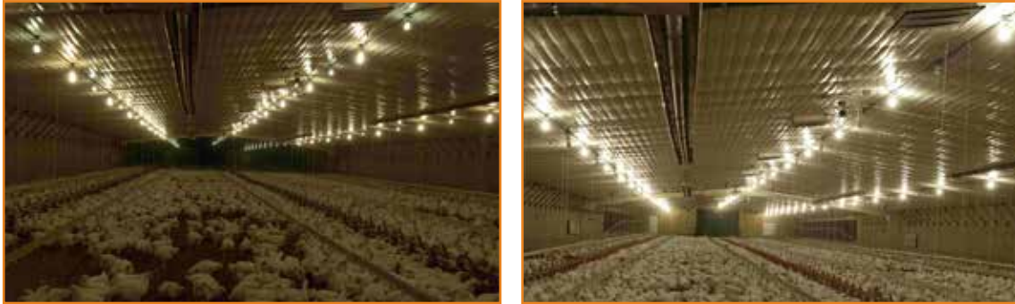
Figure 6.22: Example of 10 lux/1 fc (left hand picture) and 30 lux/3 fc (right hand picture) light intensity.
