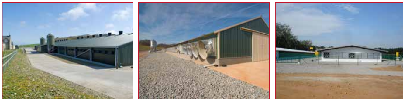
Figure 8: Houses with a low biosecurity risk showing concrete areas and no vegetation around the immediate perimeter of the house.
