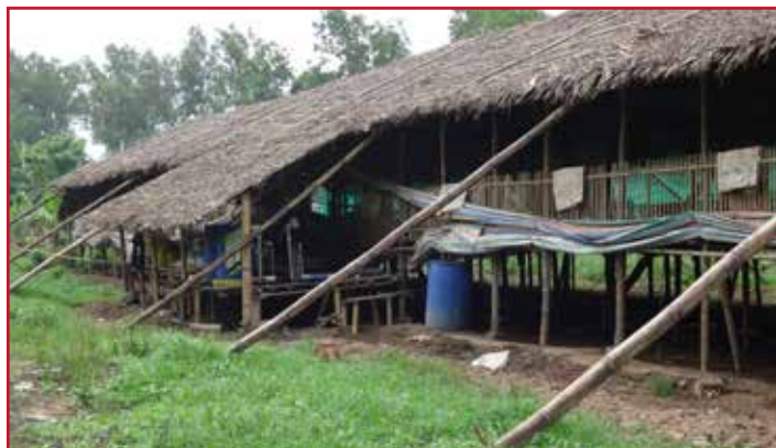
Figure 99: Example of typical open-sided housing.
