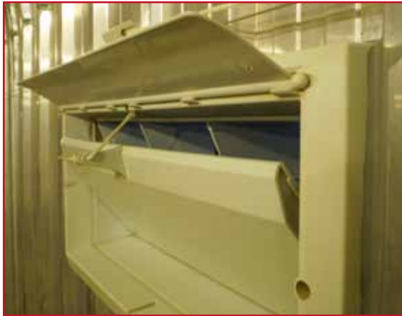
Figure 109: Example of a good-quality air inlet.
